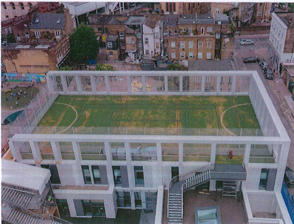
Beispiel 2: Battersea Park High School (London)
