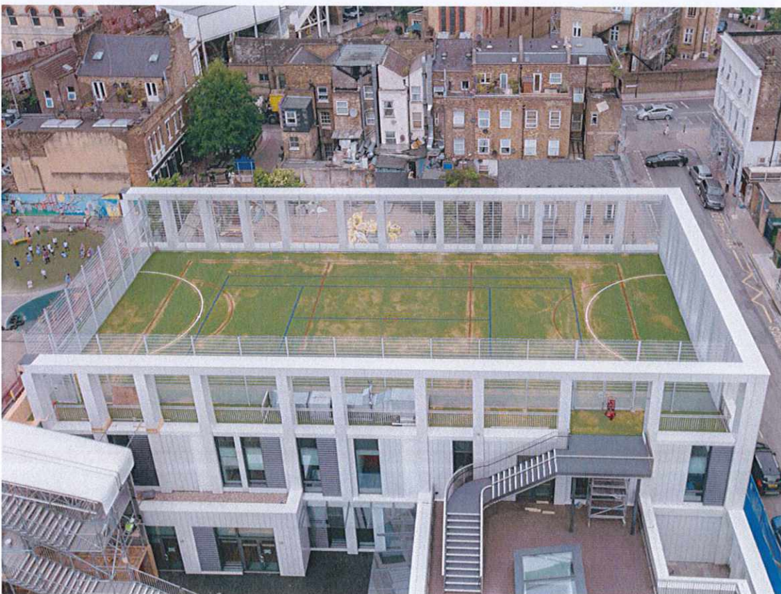
Beispiel 2: Battersea Park High School (London)
